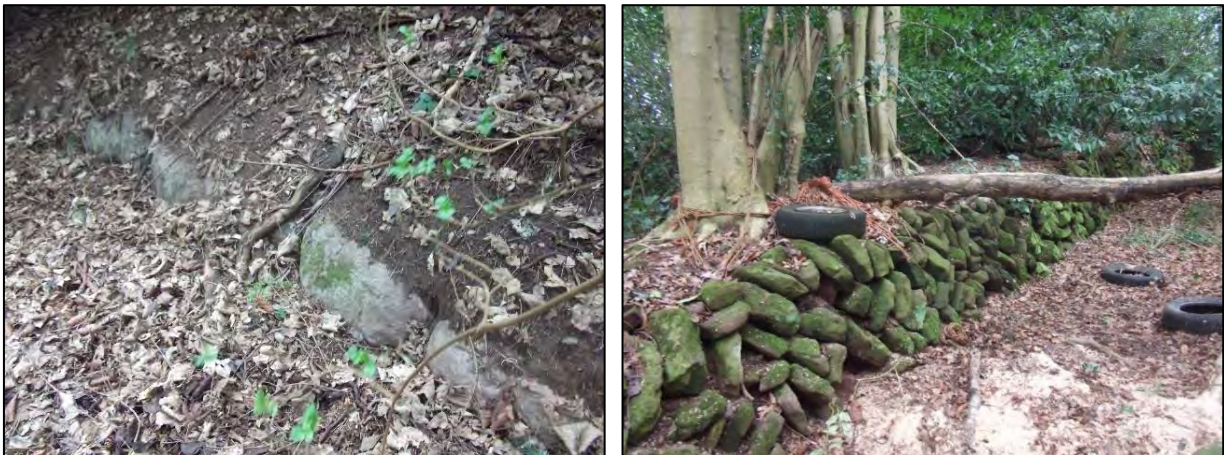
Figure 34: The boulder revetment in the Dingle (left) the stacked stone revetment forming part of one of the sunken pathways through the western part of the garden (right)
