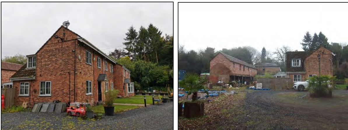
Figure 31: The converted remains of the cowshed into two domestic residences (left) and the Bottom Yard complex, showing the long barn and evidence of the raised roof on its north gable end (right)
